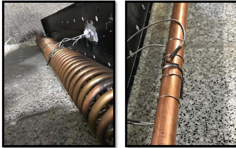
Figure (8) Locations of thermocouples for measuring water temperature surrounding the tube heat exchanger.
