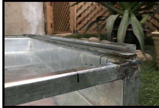
Figure (4) A close view of the base position of the glass layer in the enclosure.
