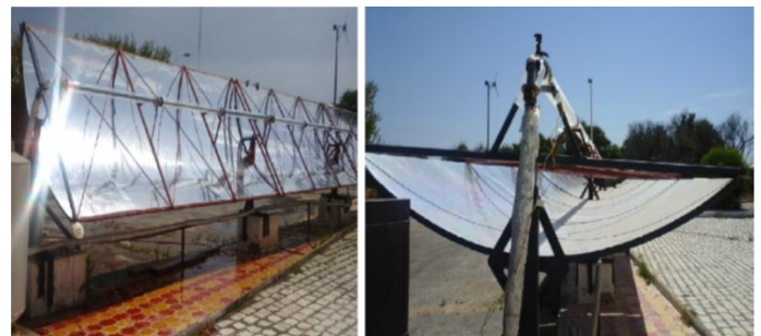
Fig.4: The Parabolic Trough Solar Collectors in two different tracking positions [36].
