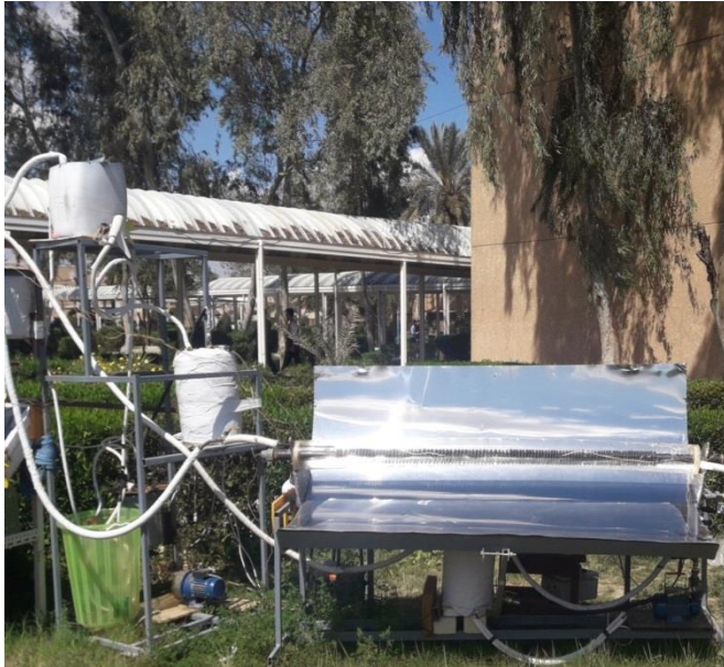
Fig. 3 Fabrication of Solar Absorption Refrigeration System.
